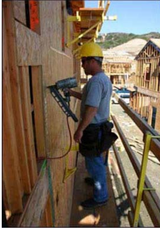
Figure 29 - A worker sheathing walls from an exterior bracket scaffold.
