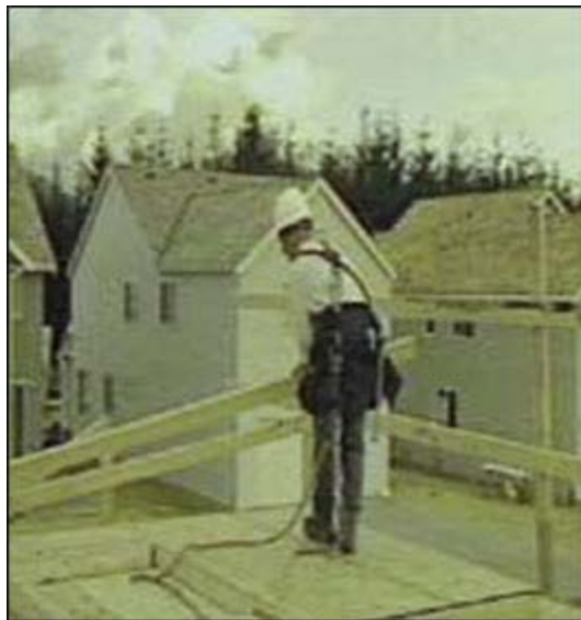
Figure 27 - Worker installing guardrails.
