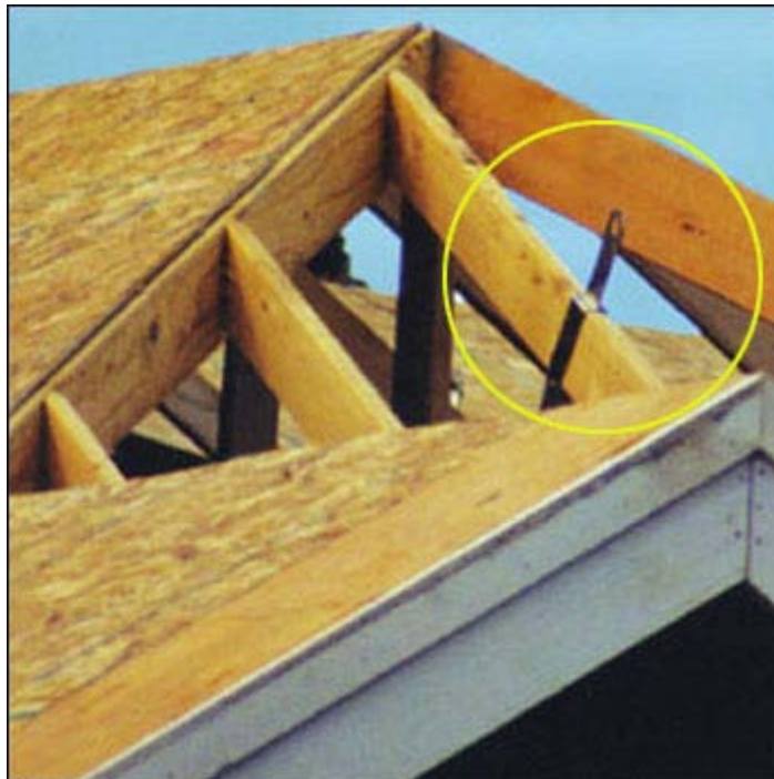
Figure 6 - A bolt-on anchor attached to a rafter.
