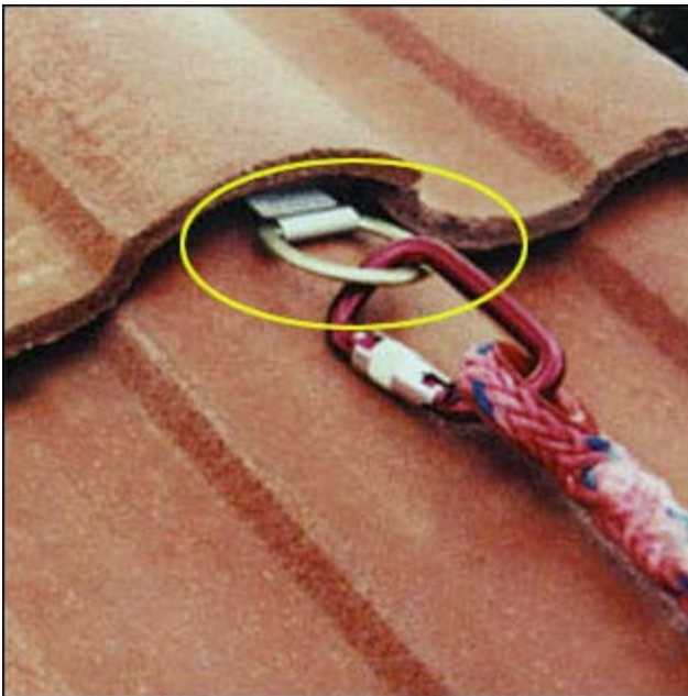
Figures 11 & 12 - Permanent anchors on completed roofs.
