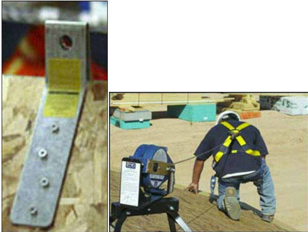
Figure 9 - Anchors that can be used while performing roof sheathing operations.
