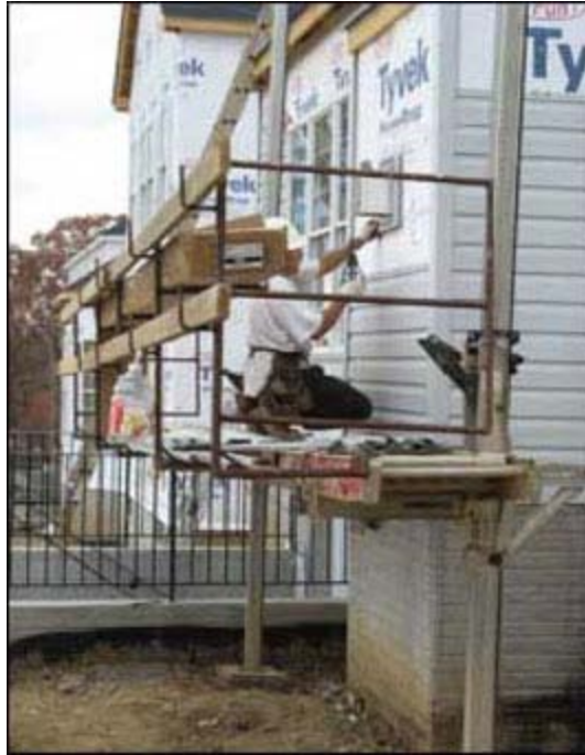
Figure 32 - A worker performing siding activities from a pump jack scaffold.
