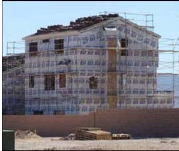
Figure 28 - Welded end frame scaffold.
