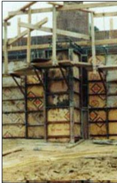
Figure 16 - A bracket-form scaffold attached to formwork.
