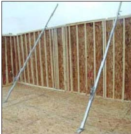
Figure 23 - Framed walls being erected using a jack.
