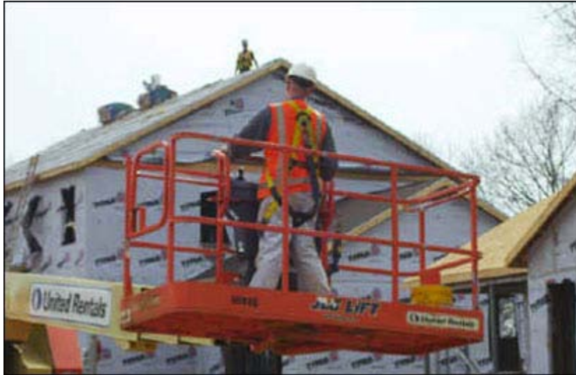
Figure 31 - Worker positioning an aerial lift.
