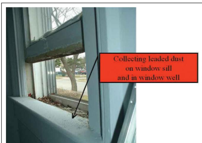
**FIGURE 5.13** Window sill (at arrow); trough is behind sill, under sash and in front of storm window tracks.
