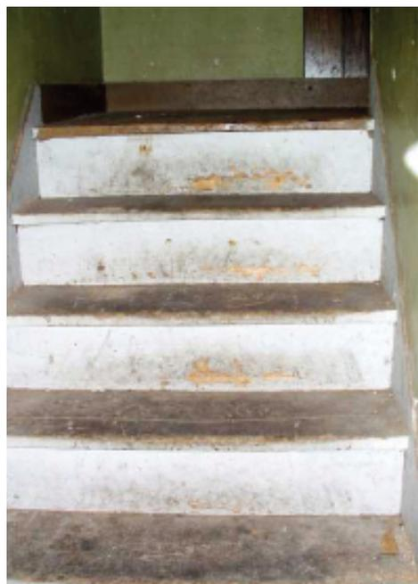
**FIGURE 5.6a** Friction hazard on stairs pre-treatment.
