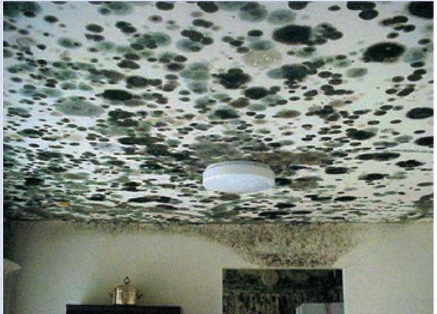
*Photo 2: Extensive mold contamination of ceiling and walls*
