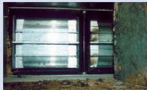
*Photo 4C: Moldy air duct*
